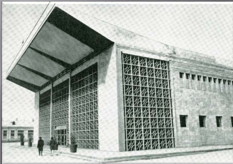
Overground lobbies of “Khatai” station
