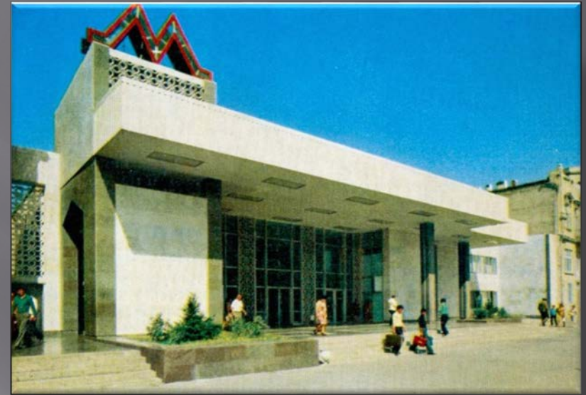
Overground lobbies of “Nizami” station
