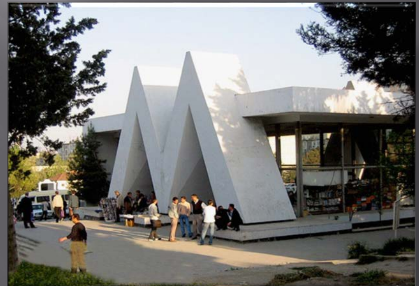
Overground lobbies of “Memar Adjemy” station
